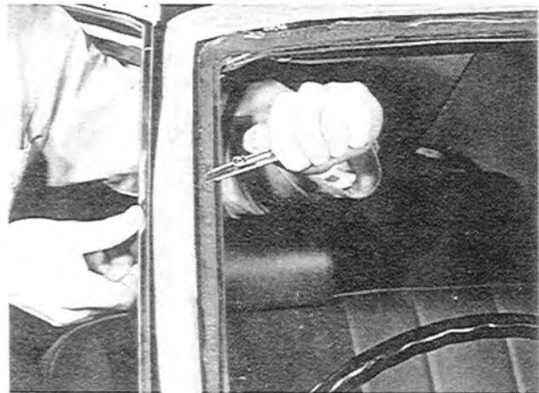
Fig. 14-7 Cutting of sealant
